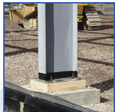
Column Base Thermal Break
